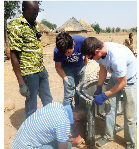
Above left: Rachel Aukamp '18 and Cheylee Smith '20 dig around the newly implemented ferro-cement liner to create a level ground surface for laying the concrete slab. Above right: Eric Denlinger '19 and Adam Barley '19 remove the ferro-cement liner from its mold.
